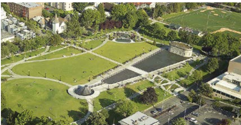
Lincoln Reservoir Cal Anderson Park SEATTLE, USA
